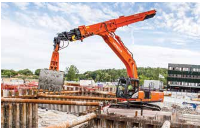
Special application excavators
